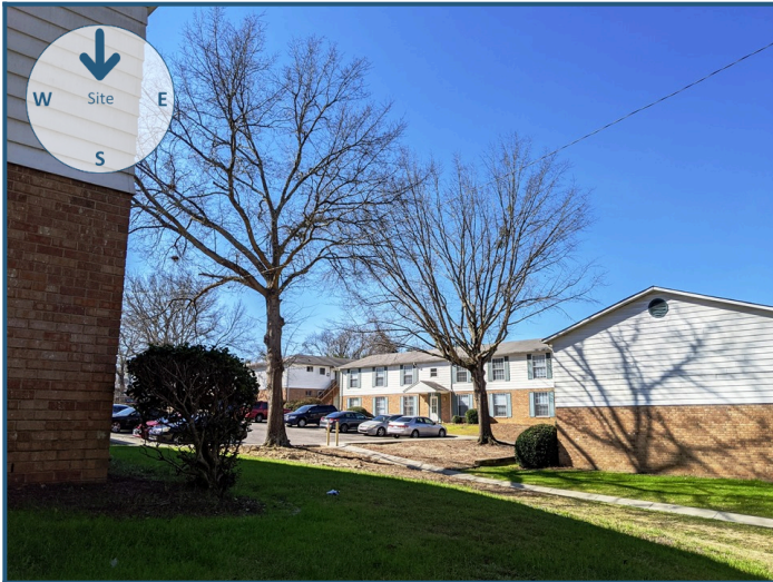
View of site from the north
