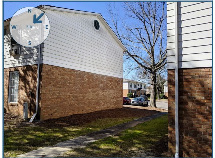
View of site from the northeast
