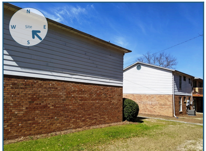
View of site from the southeast
